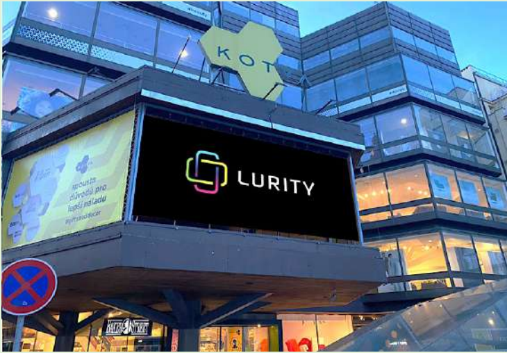
LED outdoor OC Kotva, Praha
